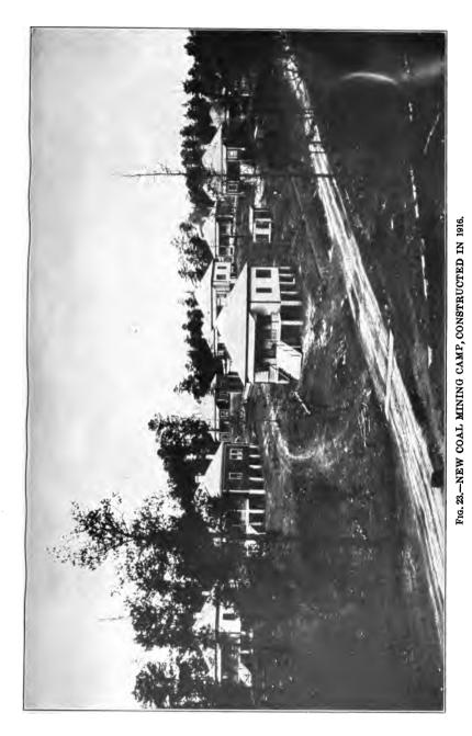
Houses built before grading and laying of streets. All cottages of similar plan and adapted for conversion into double houses. Used as one-family 4-room houses. Running water in kitchen, electric light. Ceiled inside, composition roof. Final cost \$807 (house proper, \$666; wiring, \$30; piping for water, \$45; fences, \$31; clearing site, \$10; grading streets, \$25); rent, \$6 per month.
